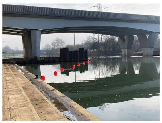
Contractors working on repairs to the Parkway Bridge have installed a coffer dam extending someway in to the river below the bridge, substantially reducing both the navigable width of the river and visibility of oncoming river
